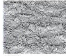
CSP 9 (heavy scarification)
